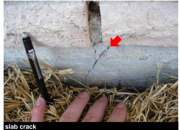
slab crack
