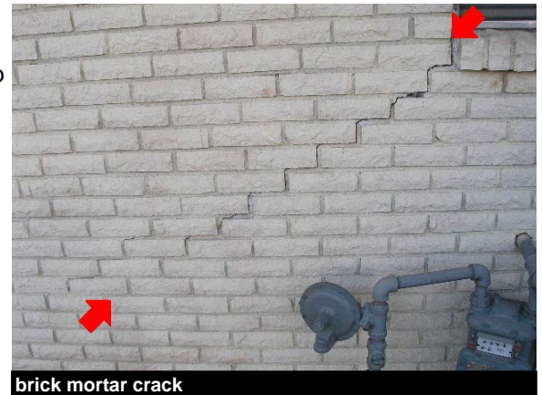
brick mortar crack
