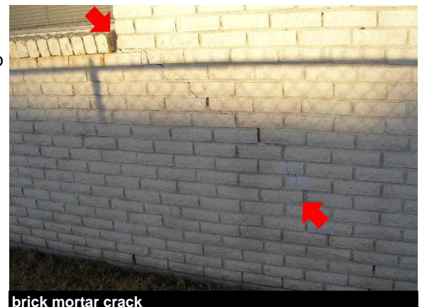
brick mortar crack
