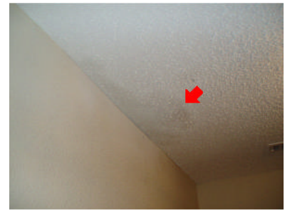
Chimney Stack Rear Bedroom Closet
